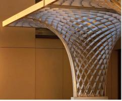
Figure 17: Asymptotic Canopy for the Intergroup Hotel in Ingolstadt. The grid is designed with a transition from 90 to approximately 60 node angles, thus allowing for a bespoke shape and a directed load-path. Each segment prefabricated hanging upside down, to form the design geometry.
