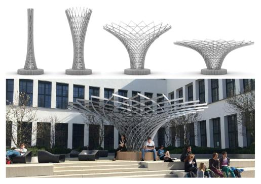
Figure 18: The Asymptotic Umbrella is a transformable structure. It is actuated by vertical cables which gradually open the angles in the upper part of the grid, causing the umbrella to unfold.
